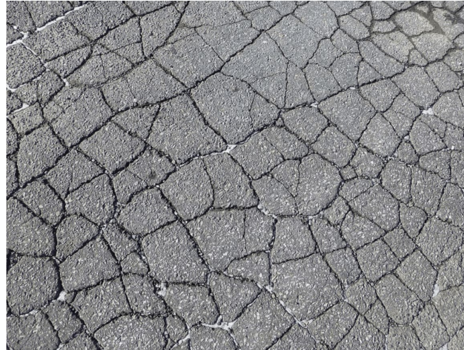
FATIGUE CRACKS
