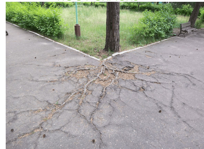
ROOT CRACKS
