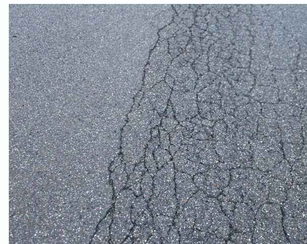
ROOT CRACKS
