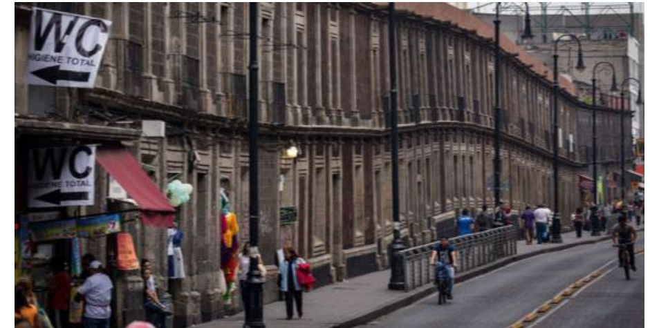
Unlevel sinking and undulating rooflines in Mexico City ( www.sciencemag.org )
