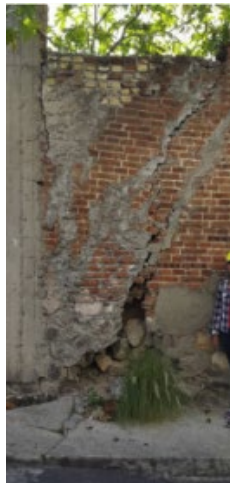
Fissuring and cracking of houses due to differential subsidence (FIGUEROA-MIRANDA et al. 2018)
