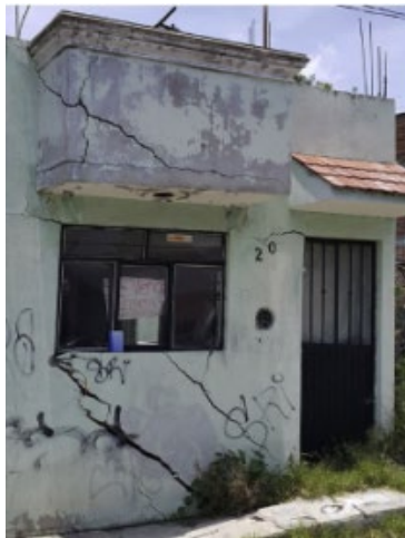
Fissuring and cracking of houses due to differential subsidence (FIGUEROA-MIRANDA et al. 2018)
