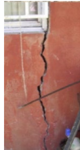
Fissuring and cracking of houses due to differential subsidence (FIGUEROA-MIRANDA et al. 2018)
