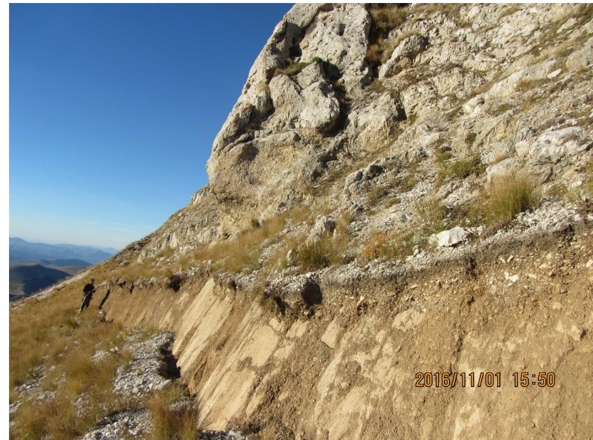
Normal fault offset in 2016 Central Apennines, Italy earthquakes (from Laura Gregory)
